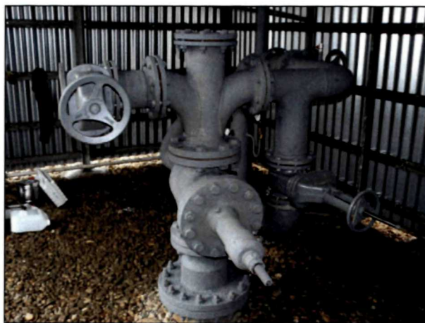
Fig. 4.8 Reinjection well in Podhájska GRP-1 (Photo: D. Marcin, 2012)
